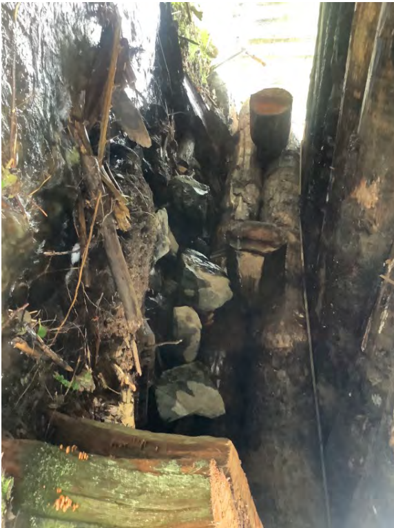
Right Bank Abutment when facing downstream
