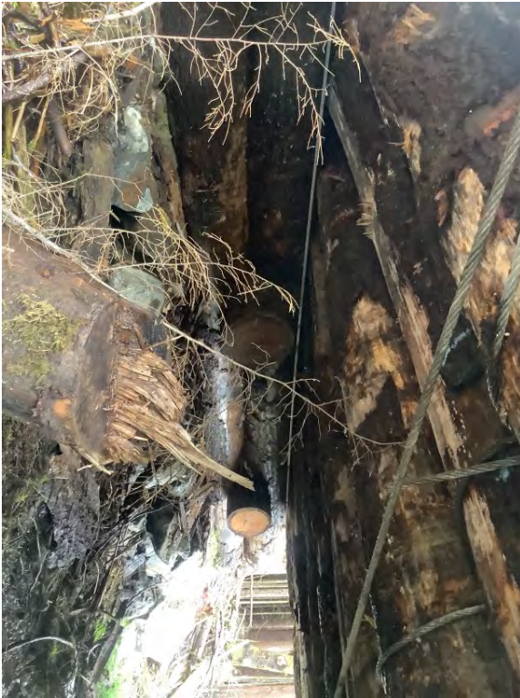
Left Bank Abutment when facing downstream
